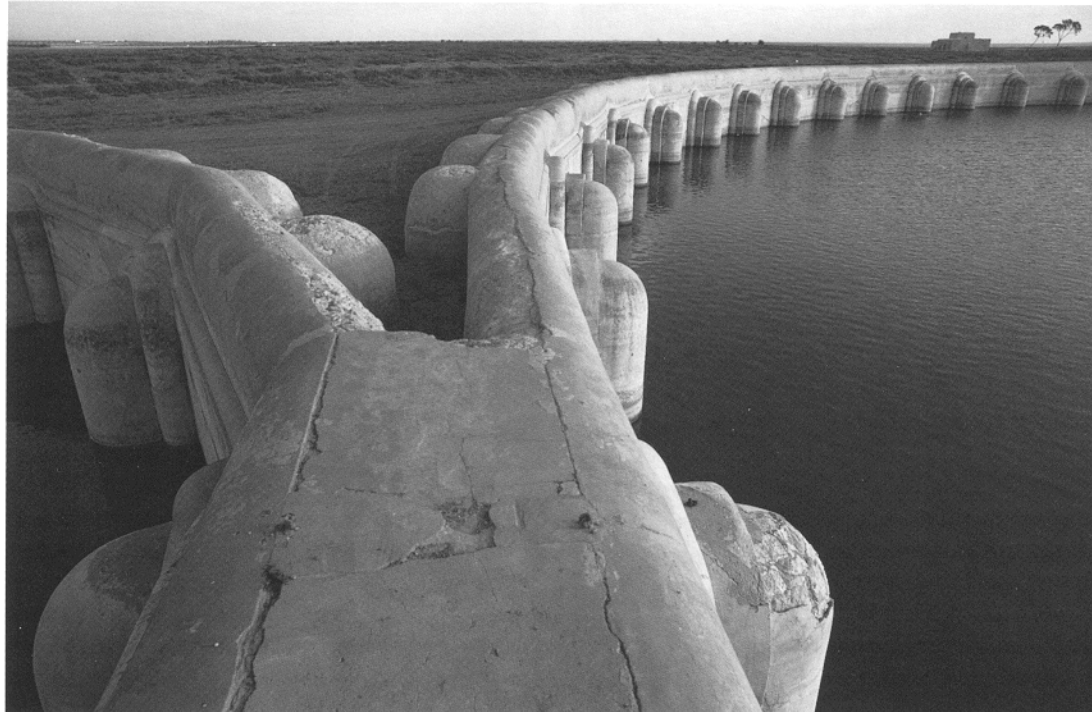
This dam in Tunisia is centuries old and still functioning. Like several other dams built throughout the Islamic world, it displays remarkable technological knowledge including the use of the correct curvature needed to offer the maximum resistance to the pressure of the water.
